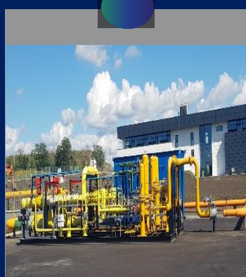
Lucrari de instalatii in constructii
