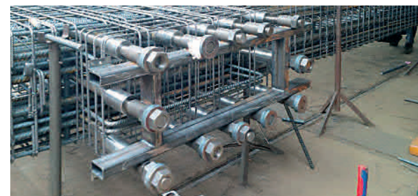
COPRA Anchoring Couplers in a double-sided beam-to-column connection
